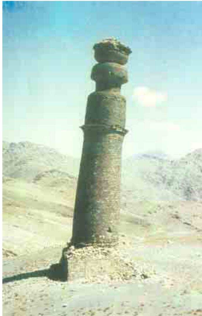
Ilus.1 the column tilted some 4 degrees to the south
