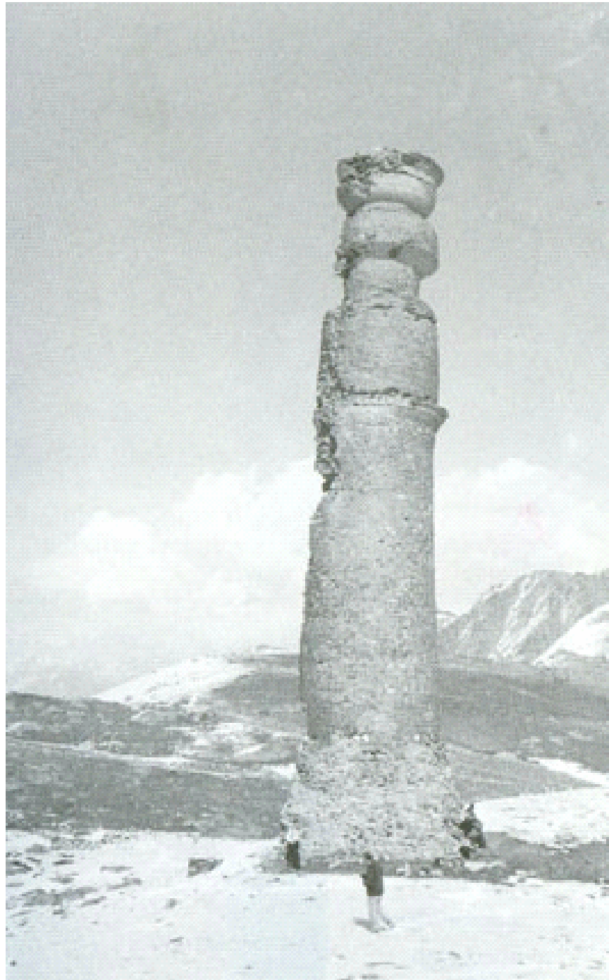
Il lus. 4 in the 1980s the column was damaged by shelling
